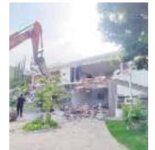
HYDRAA conducting demolitions at Gandipet FTL lands on Sunday
