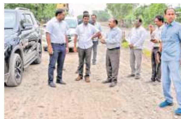
Peddapalli Collector Koyad Sri Harshad inspecting road repair works in Ramagundam on Tuesday
