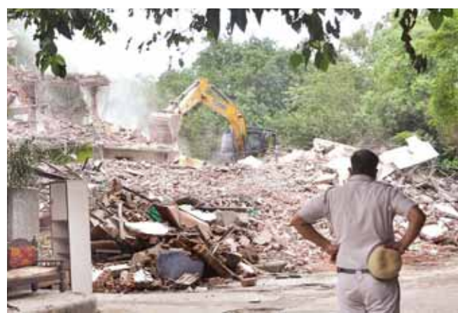
A police personnel during a demolition drive at Khyber Pass area, in New Delhi, on Sunday Ranjan Dimiri/Pioneer
