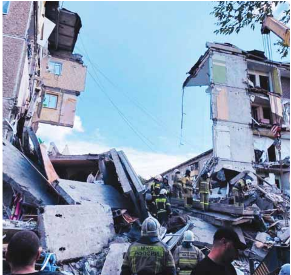
In this photo released by the Telegram channel of the head of Nizhny Tagil Vladislav Pinyavov on Thursday, August 1, 2024, Russian Emergency Ministry workers are seen near a multi-storey building partially collapsed presumably due to gas explosion in Nizhny Tagil, 1400km (870mi) east from Moscow, Sverdlovsk region, Russia. Three people have reportedly been rescued from under the rubble, information about the victims is being clarified. AP/PTI
