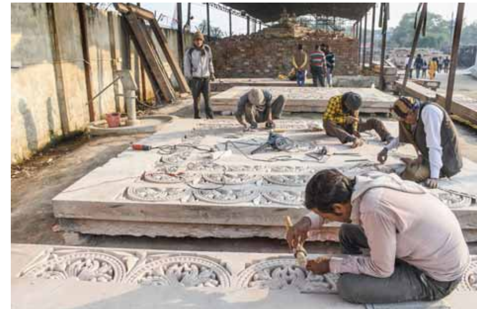
A worker carves stone as part of construction of Ram Temple, in Ayodhya on Sunday
