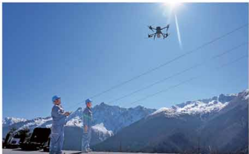
The staff were using the drone to patrol power transmission lines in Yunnan. (Photo by Yunnan Daily)
