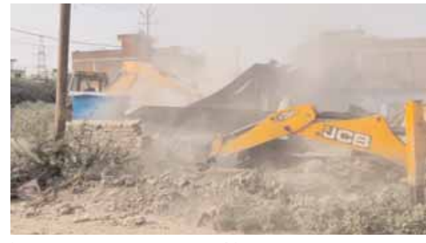
Illegal construction being demolished by KDA enforcement squad.
