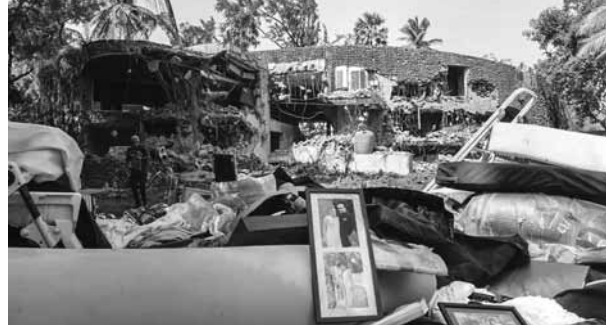
A view of Nirav Modi's demolished bungalow in Alibaugh town near Mumbai on Friday
