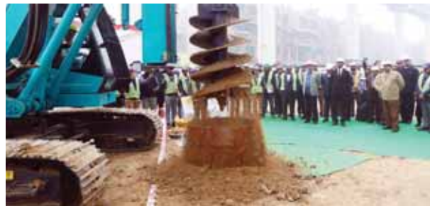
PHASE IV CONSTRUCTION WORK BEGINS
